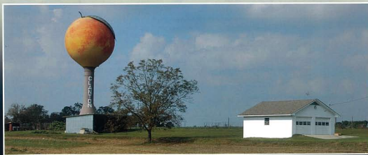
FRUIT FIGHT: The peach water tank in Canton, Alabama, is a smaller—if not quite bite-sized—version of the Peachoid.
